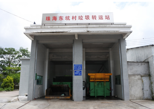
Dongkengchuan Refuse Transfer Station 东坑村垃圾中转站
