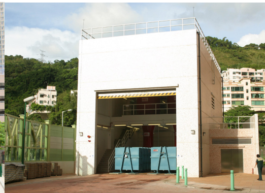
Tseung Kwan O Choi Ming Court Refuse Transfer Station 将军澳彩明苑中央收集站
